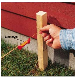
**4** Attach a line level to one of the mason's strings to use as a reference. Adjust the string up or down as necessary until it is level. Adjust the other strings until they are level, making sure that intersecting strings contact one another (this ensures that they are all at the same height relative to ground level).
