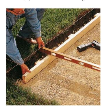
**4 Drive 3" Deck Screws** through the stakes and into the form board on one side. Set a level so it spans the staked side of the form and the opposite form board, and use the level as a guide as you stake the second form board so it is level with the first. For large projects, use the mason's strings as the primary guide for setting the height of all form boards.
