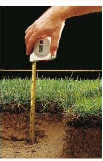
**2 Dig a test hole** to the planned depth so you can evaluate the soil conditions and get a better idea of how easy the excavation will be. Sandy or loose soil may require amending; consult a landscape engineer.
