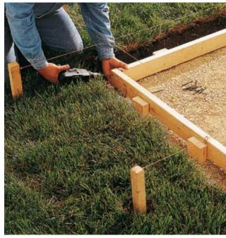
**5** Once the forms are staked and leveled, drive 3" deck screws at the corners. Coat the insides of the forms with vegetable oil or a commercial release agent so concrete won't bond to them. Tip: Tack nails to the outsides of the forms to mark locations for control joints. See page 14 for joint placement recommendations.
