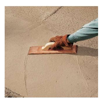
**3** Float the concrete surface to create a surface that is both smooth and skid resistant. Wait until bleed water has disappeared before proceeding. Finish options include a broomed finish, a smooth steel-trowel finish or seed with small aggregate after floating.
