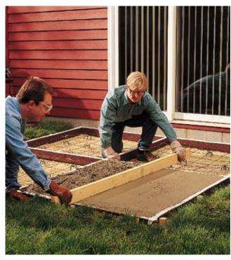
**2** Screed concrete level with the forms. Use a 2 x 4 in a sawing motion to level and remove excess concrete.
