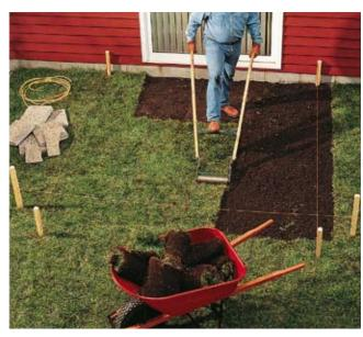
**6** Start excavating by removing the sod. Use a sod cutter if you wish to reuse the sod elsewhere in your yard (lay the sod as soon as possible). Otherwise, use a square-end spade to cut away sod. Strip off the sod at least 6" beyond the mason's strings. The subbase should extend at least 6" beyond the project area. You may need to remove the strings temporarily for this step.
