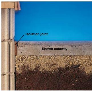
**4** When pouring concrete next to structures, glue a ½"-thick piece of asphalt-impregnated fiber board to the adjoining structure to keep the concrete from bonding with the structure. The board creates an isolation joint, allowing the structures to move independently, minimizing the risk of damage. ◆
