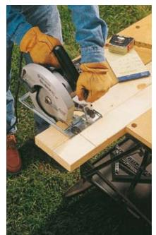
**1** • A form is a frame, usually made from  $2 \times 4$  lumber, laid around a project site to contain poured concrete and establish its thickness. Cut  $2 \times 4$ s to create a frame with inside dimensions equal to the total size of the project.
