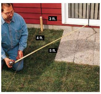
**2** Connect the stakes with mason's strings. The strings should follow the actual project outlines. To make sure the strings are square, use the 3-4-5 triangle method (see page 149): measure and mark points 3 ft. out from one corner along one string, and 4 ft. out along the intersecting string at the corner. Measure between the points, and adjust the positions of the strings until the distance between the points is exactly 5 ft. A helper will make this easier.
