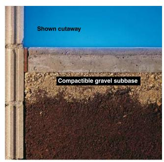
**3** Add a compactible gravel subbase to provide a level, stable foundation for the concrete. The compactible gravel also improves drainage—an important consideration if you are building on soil that is high in clay content. For most building projects, pour a layer of compactible gravel about 5" thick, and use a tamper to compress it to 4".
