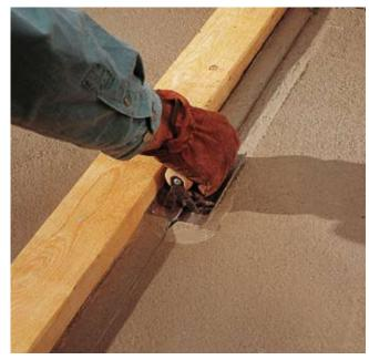
**4** ■ **Cut control joints** in larger patios. Lay a 2 x 4 straightedge guide on the surface and carefully tool control joints using a grooving tool. Allow the concrete to dry until sheen disappears, and then treat with acrylic cure and seal (see page 15). ◆
