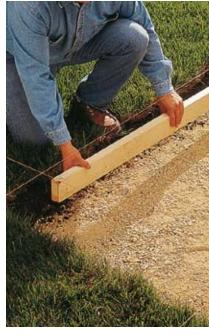
Use the mason's strings that outline the project as a reference for setting form boards in place. Starting with the longest form board, position the boards so the inside edges are directly below the strings.
