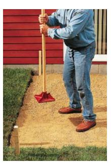
**8** Lay a subbase for the project (unless it requires a frost footing). Pour a 5"-thick layer of gravel, and tamp until the gravel is even and compressed to 4" in depth. ◆
