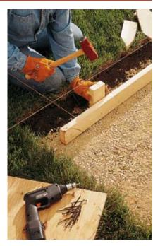
**3** Cut several pieces of 2 × 4 at least 12" long to use as stakes. Trim one end of each stake to a sharp point. Drive the stakes at 3-ft. intervals at the outside edges of the form boards, positioned to support any joints in the form boards.
