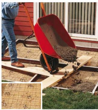
Imstall reinforcement (optional) such as rebar and rewire set on bolsters (inset photo), and then mix and pour the concrete (see pages 12 to 15 and 138 to 143). The use of fiber-reinforced crack-resistant concrete eliminates the need for wire reinforcing mesh.
