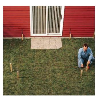
**3** Reset the stakes, if necessary, to conform to the positions of the squared strings. Check all corners with the 3-4-5 method, and adjust until the entire project area is exactly square. This can be a lengthy process with plenty of trial and error, but it is very important to the success of the project, especially if you plan to build on the concrete surface.
