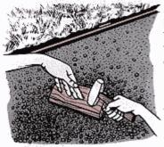
Medium-sized aggregate (including pebbles, small gravel, and seashell fragments) can be hammered into fresh concrete. Use a screed to evenly distribute the force of each blow.
