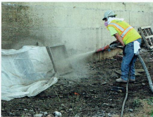
Fig. 1: Field test panel being properly gunned on site
