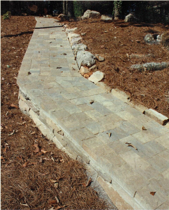
The uphill side of the walkway was lined with natural stone and boulders to inhibit erosion.
