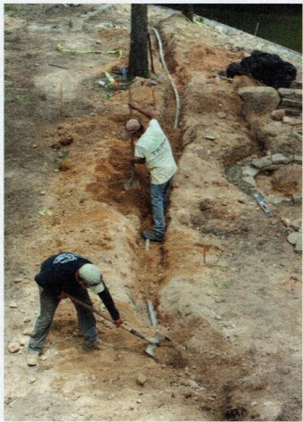
Burying the electrical line was a two-man job.
