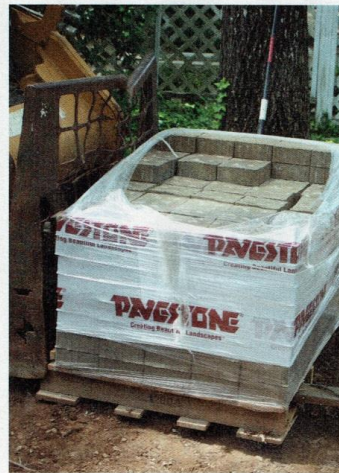
A heavy pallet of pavers requires powered equipment to move place to place.
