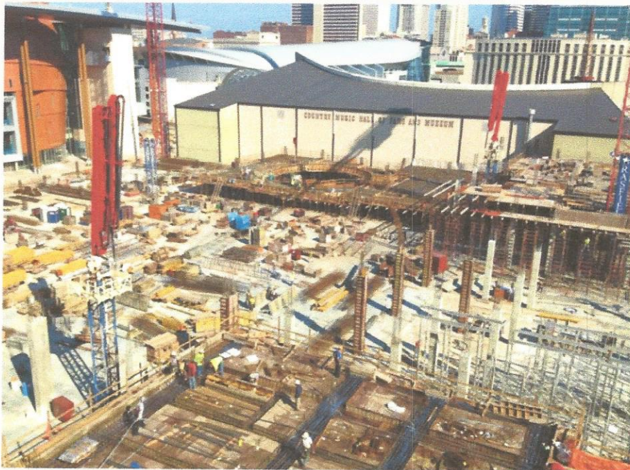
Below Bottom: Brick in the kitchen of the Omni
