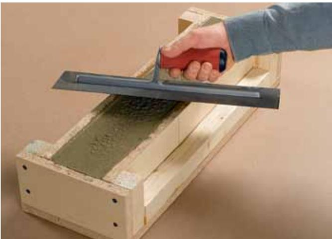
6. Screed or trowel the concrete so it is flat and flush with the top of the mold. Cover the mold with plastic sheeting and let it cure undisturbed for 48 hours.
