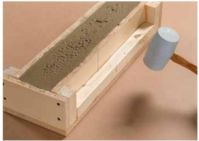
5. Fill the mold with concrete. Settle the pour into the mold by pounding the work surface with a mallet or lifting the corners of the mold and tapping it onto the work surface.
