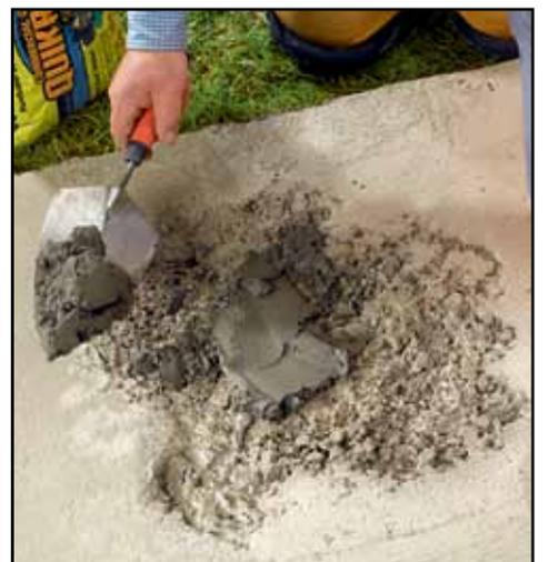
The repair material should be built up in layers with the first layer being pressed into the repair area with firm trowel pressure.
