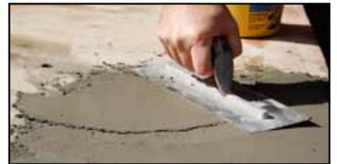
For repairs to concrete edges and corners QUIKRETE® Quick-Setting Cement should be used along with QUIKRETE® Acrylic Fortifier. Quick-Setting Cement can be molded and shaped to match the surrounding contour of the concrete and sets in about 10 minutes. Acrylic Fortifier provides the bond strength necessary for a long-lasting repair.
