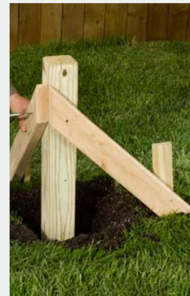
**3 ■ Set the post** in the hole. Attach angled 2 x 4 braces to two adjacent sides of the post using one screw for each brace. Drive a stake into the ground near the lower end of each brace.
