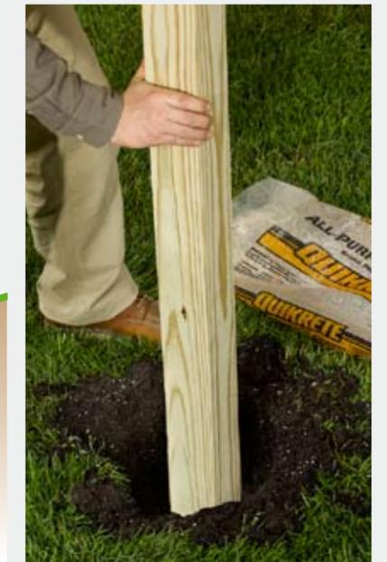
**1 ■ Dig the post hole**, making it three times the width of the post and at a depth equal to  $\frac{1}{3}$  to  $\frac{1}{2}$  of the above-ground length of the post, plus 6" (right). For loose or sandy soil, using a tube form is recommended (left).
