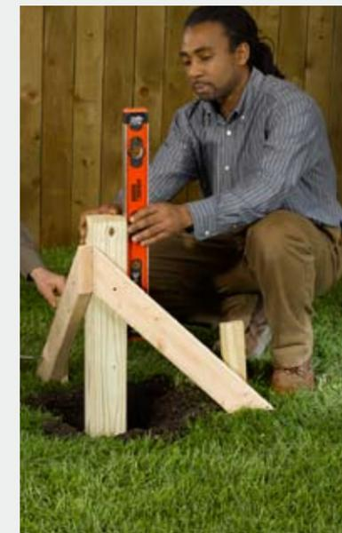
**4 ■ Use a level** to position the post plumb (perfectly vertical), checking on two adjacent sides using one screw for each brace. Drive a stake into the ground near the lower end of each brace.
