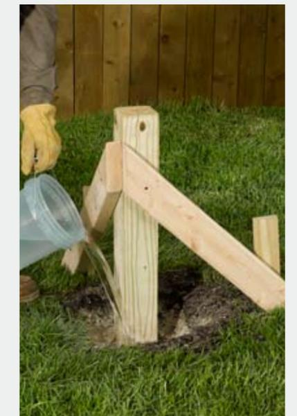
**5 ■ Fill the hole** with concrete up to 3 to 4" below the ground level. Add the recommended amount of water. After the concrete has set, backfill the hole with soil and/or sod.
