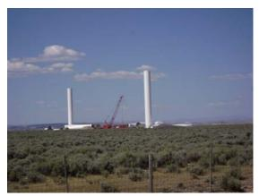
By design, the base of a wind turbine takes the brunt of the high torque generated as the massive turbine is spun by the wind. Without a strong grout supporting the pedestal, the turbine could be at risk for structural failure.
