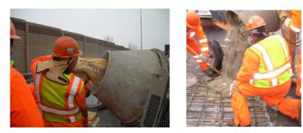
Construction crews are primarily using QUIKRETE<sup>®</sup> FastSet<sup>™</sup> DOT Mix – Extended and QUIKRETE<sup>®</sup> FastSet<sup>™</sup> DOT Mix for roadway and bridge deck patching and full-depth repairs to reinforce the structural steel reinforcement bars (rebar). QUIKRETE<sup>®</sup> FastSet<sup>™</sup> DOT Mix was selected due to its consistency and workability; setting in approximately 30 minutes and reaching a compressive strength of 4,500 pounds-per-square-inch in three hours.
