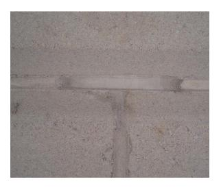
Leading edge discoloration of a mortar patch – over tooling
