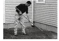
**2.** Remove the sod and soil to the desired depth. Remember to account for the width of the forming lumber.
