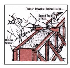
7. Depending on the amount of concrete to be poured and the people available to do the job, it might be necessary to construct the wall in sections by using a movable stop board. Drill holes through the stop board so that it can be moved along the wall without cutting the rebar.
