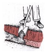
**6.** If the footer is to be the base of a poured concrete wall, install a keyway form as shown. This keyway will help tie together the footer and wall.
