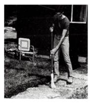
**3.** Set and stake forms against the old sidewalk or slab. Backfill against the forms to ensure sufficient support.
