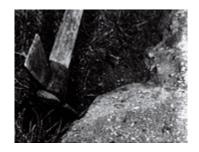
**2.** Remove all broken and loose concrete, dirt, dust and plant remains to form a sound base for the new topping. Use QUIKRETE® Concrete & Asphalt Cleaner to remove dirt or grease stains.
