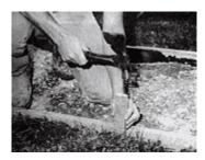
**4.** Use a level to make sure that the forms are set at the correct height and that there is adequate slope drainage.
