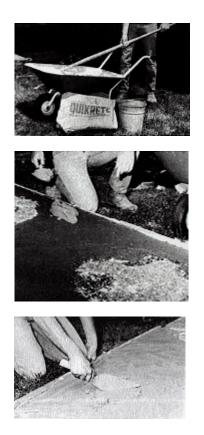
**7.** Trowel the surface smooth using a steel finishing trowel. Edge using a concrete edger if desired.
