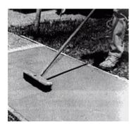
**9.** Cure the new surface with QUIKRETE® Acrylic Concrete Cure & Seal. Apply after finishing when surface sheen has disappeared and
