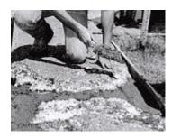
**4.** The final 1" topping is made of QUIKRETE® Sand Mix. When this layer is less than 1", add QUIKRETE® Concrete Acrylic Fortifier as part of the Sand Mix liquid. Note: For Sand Mix toppings thicker than 1", but less than 2", do not use Acrylic Fortifier. Instead, apply QUIKRETE® Concrete Bonding Adhesive. In this job, the concrete mix patch separates the adhesive and fortified sand mix.
