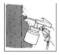
**3.** Apply the QUIKWALL® SBC in the same manner as described earlier. When relining silos, it is very important that the walls be troweled extra smooth to minimize the occurance of small pockets where future acid crusting could originate.
