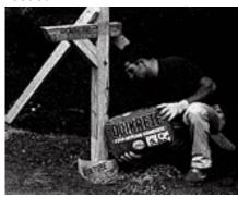
**5.** Pour water onto the dry mix and allow it to soak in. Depending on soil conditions, you will need about 1 gallon of water for each 50lb. bag of Fast-Setting Concrete Mix placed in the hole. Dig larger, dish-shaped holes for posts set in loose or sandy soil.
