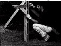
**4.** Pour the Fast-Setting Concrete Mix dry from the bag into the hole until it reaches 3" to 4" (100mm) from the top. Recheck the post for plumb and brace as needed.
