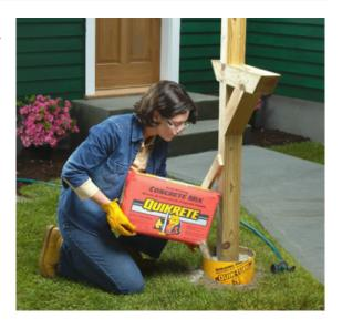
For heavy load-bearing applications, use QUIKRETE® Fast-Setting Concrete and QUIK-TUBE™ Building Forms.
