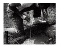
**4.** Butter the head joints of the stones before setting them in place. Once the first course has been laid, spread a layer or mortar on top of the stones and begin laying the second course.
