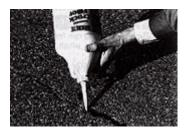
**3.** For deep cracks, sprinkle clean sand into the crack within  $\frac{1}{4}$ " of the surface before applying the Crack Seal.
