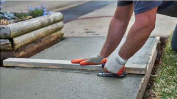
Use a groover and straight-edge to cut in control joints. Control joints are designed to allow for expansion, contraction and movement of the concrete slabs. 4" thick slabs require control joints a minimum of every 10 lineal feet. The control joint must be cut a minimum of 1/4 the depth of the slab.
