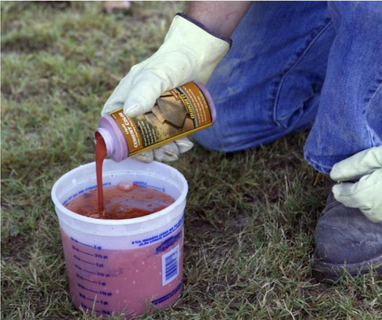
*For a uniform mix, add liquid cement color to the mixing water, before mixing the concrete.*
