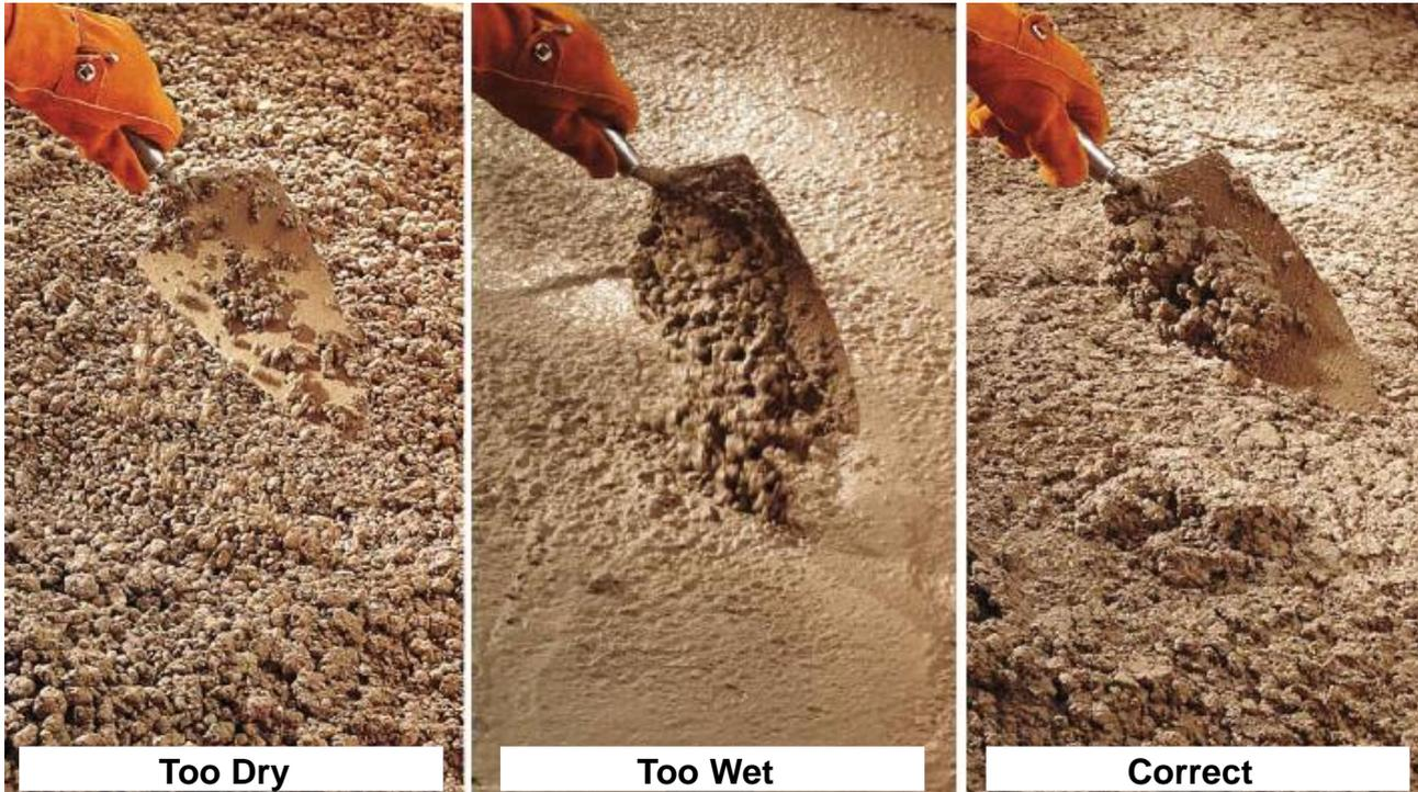
When mixing concrete, it is important to know that **the more water that is added to the mix, the weaker the concrete becomes.** Concrete is designed to reach specific minimum compressive strengths, based on the water addition instructions listed on the bag.
