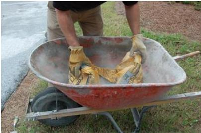
**Hand mixing** can be done in a mortar tub or wheelbarrow with a shovel or hoe.
