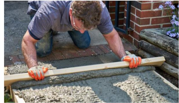
Once the concrete has lost its sheen (the bleed water has evaporated) use a wood float in an arching motion to smooth the concrete surface.
