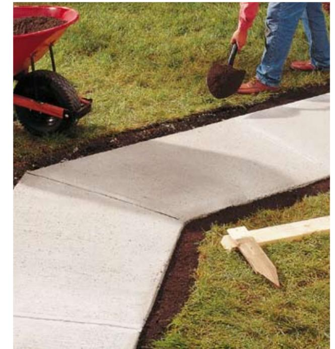
**14 ■ Remove the forms, then backfill the space** at the sides of the walkway with dirt or sod. ♦
