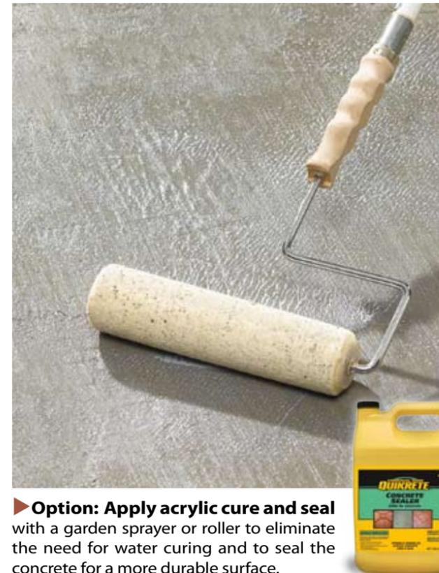
► **Option: Apply acrylic cure and seal** with a garden sprayer or roller to eliminate the need for water curing and to seal the concrete for a more durable surface.
