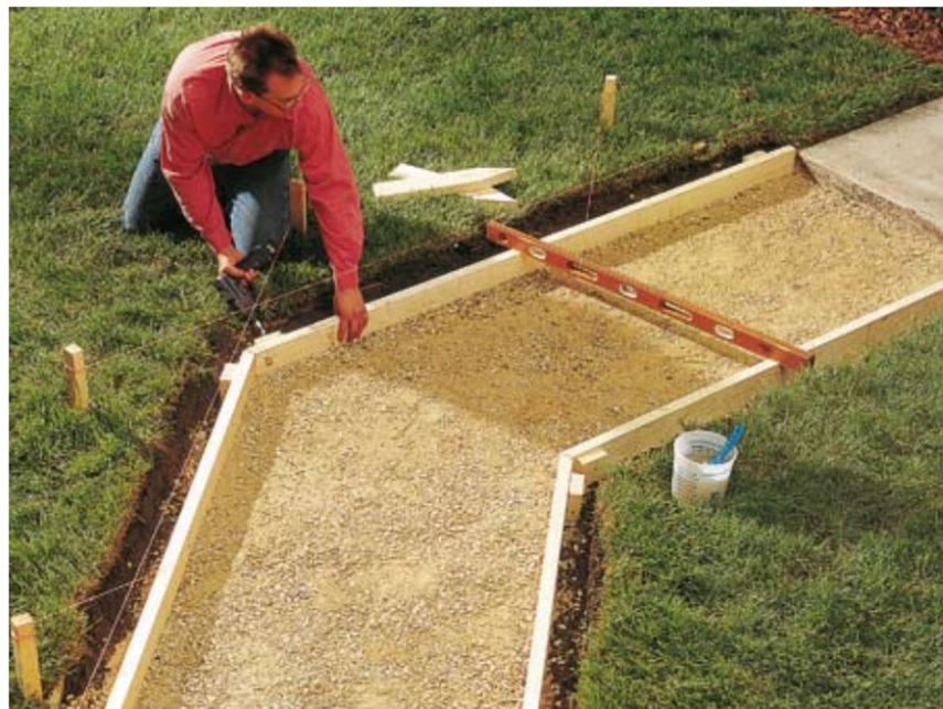
**3 ■ Build and install 2 x 4 forms set on edge.** Miter-cut the ends at angled joints. Position them so the inside edges are lined up with the strings. Attach the forms with 3" deck screws, then drive 2 x 4 stakes next to the forms at 3-ft. intervals. Attach the stakes to the forms with 2½" deck screws. Use a level to make sure forms are level or set to achieve the desired slope. Drive stakes at each side of angled joints.
