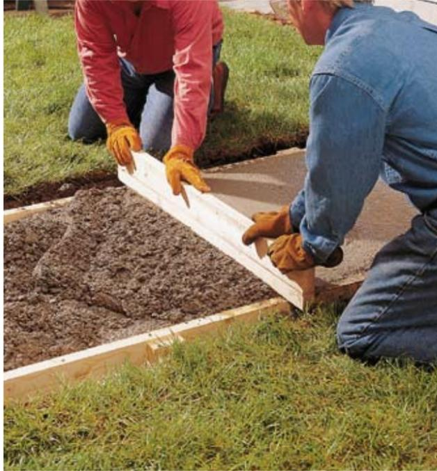
**8 ■ Build a curved screed board** and use it to form a crown when you smooth out the concrete. Note: A helper makes this easier.
