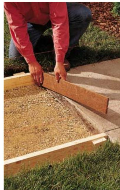
**4 ■ Glue an isolation board** to the steps, house foundation, or other permanent structures that adjoin the walkway using construction adhesive.
