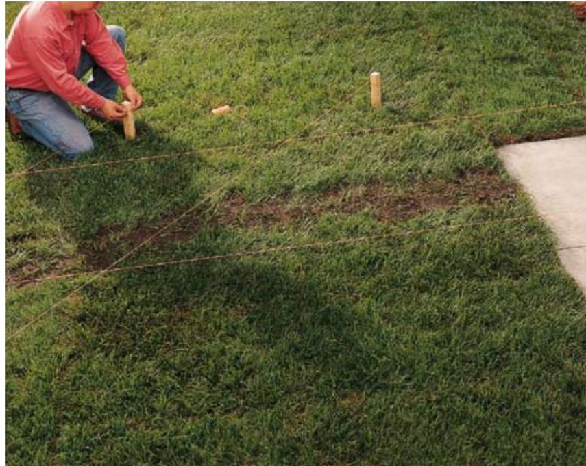
**1 ■ Select a rough layout, including any turns.** Stake out the location and connect the stakes with mason's strings. Set the slope, if needed. Remove sod between and 6" beyond the lines, then excavate the site with a spade to a depth 4" greater than the thickness of the concrete walkway, following the slope lines to maintain consistent depth.
