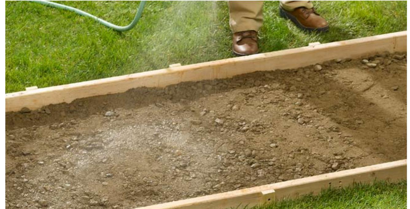
**5 ■ Prior to placing concrete,** it is necessary to dampen the gravel subbase. Spray the subbase using a water hose until saturated but do not leave standing water.
