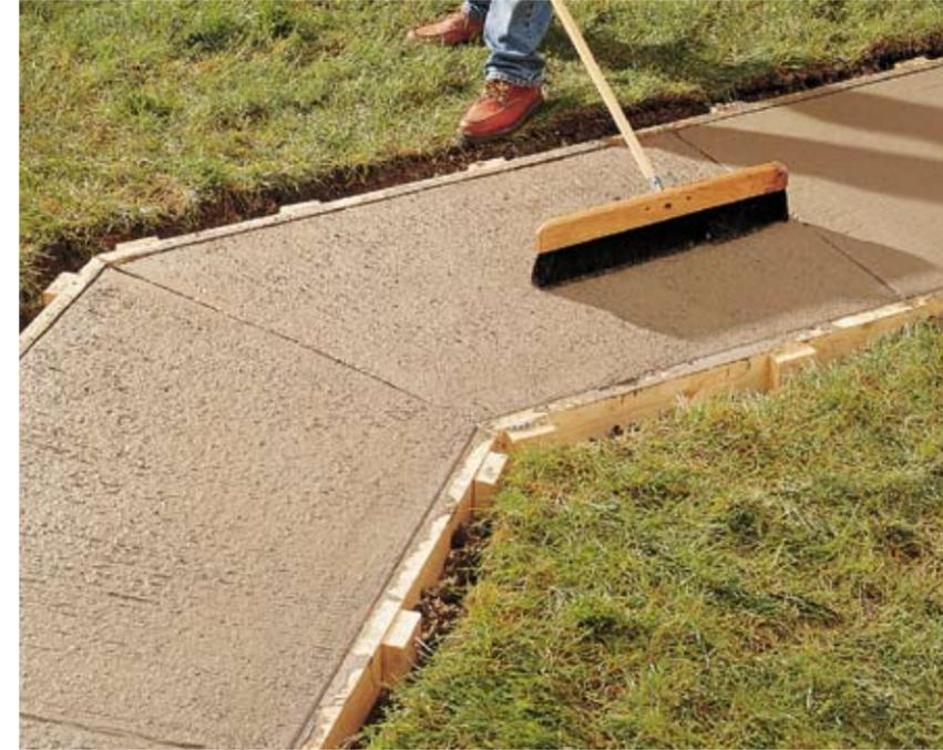
**12 ■ Create a textured, nonskid surface** by drawing a clean, stiff-bristled broom across the surface once the surface is thumbprint hard. Avoid overlapping broom marks.
