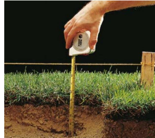
■ **Install stakes and strings** when laying out straight walkways, and measure from the strings to ensure straight sides and uniform excavation depth.
