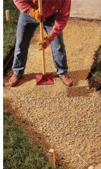
**2 ■ Pour a 5" layer** of compactible gravel as a subbase for the walkway. Tamp the subbase until it compacts to an even 4"- thick layer.
