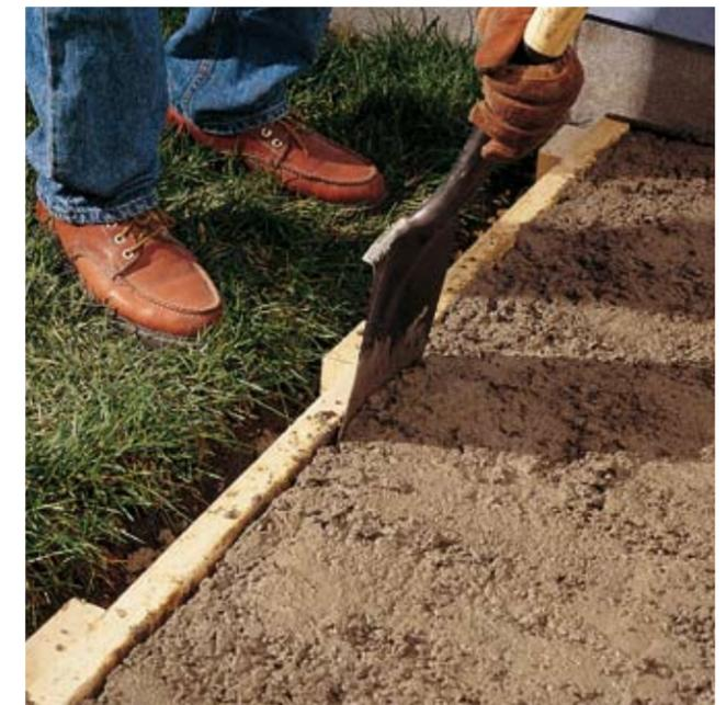
**7 ■ After pouring all of the concrete,** run a spade along the inside edges of the form, then rap the outside edges of the forms with a hammer to help settle the concrete.
