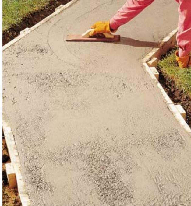
**9 ■ Smooth the concrete surface** with a wood float. The goal is to smooth it, not to level it (you should maintain the slight crown created by the curved screed board).
