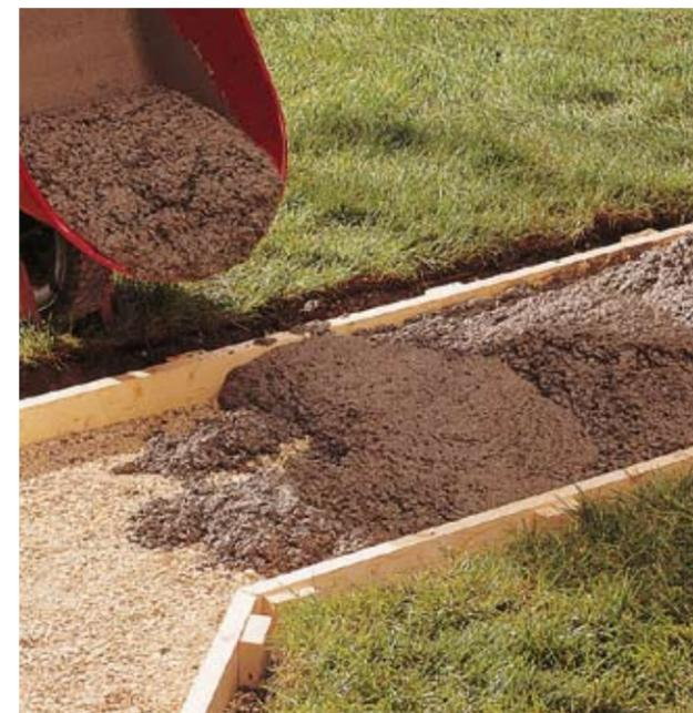
**6 ■ Mix, then pour concrete** into the project area. Use a masonry hoe to spread it evenly within the forms.
