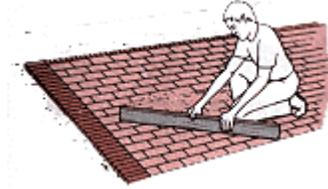
4. Spread All-Purpose Sand over the repaired area and sweep it into the joints. Dampen the sand with a fine spray; repeat until the joints are completely filled.
