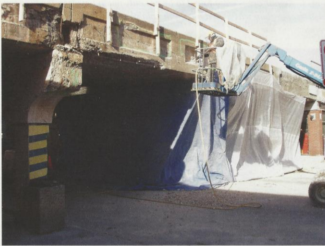
Fig. 4: Heated enclosures were installed on portions of bridge during winter months
