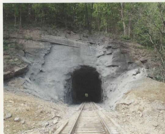
Fig. 7: West portal—final liner
