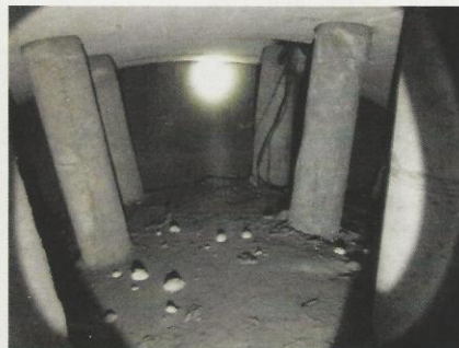
Fig. 6: Embedded hangers in existing void space between main tunnel and ventilation arch wall
