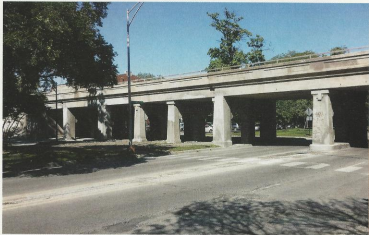
Fig. 2: Repaired 11 piers spanning 250 ft (76.2 m) over six lanes of traffic
