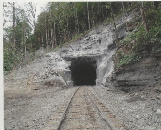
Fig. 8: East portal—final liner
