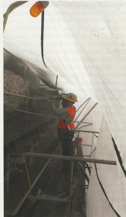
Fig. 6: Shotcrete placement inside a heated bridge enclosure
