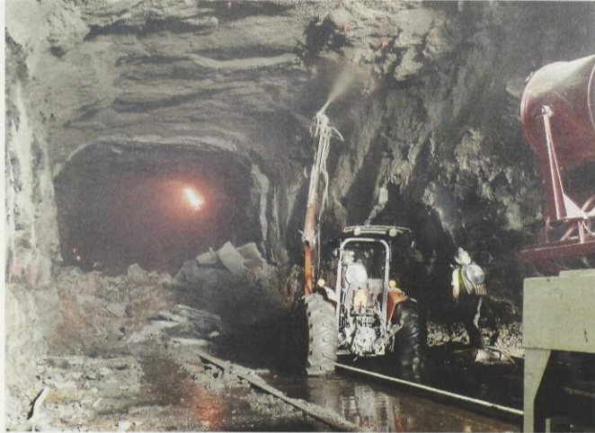
Fig. 2: Initial shotcrete roof support
