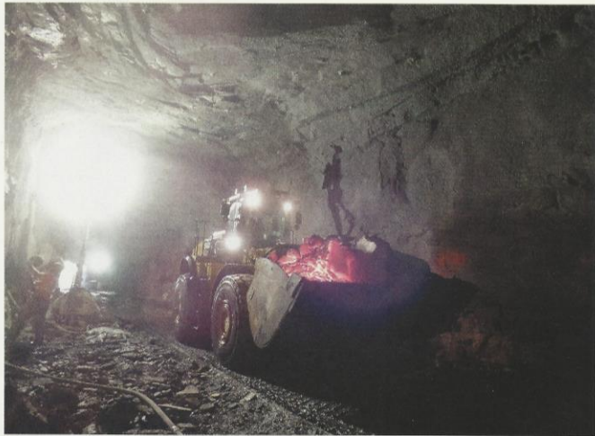
Fig. 3: Muck removal with loader
