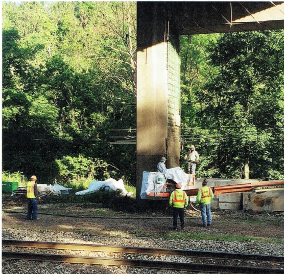
Material being cut and finished to match the original shape and profile of the pier
