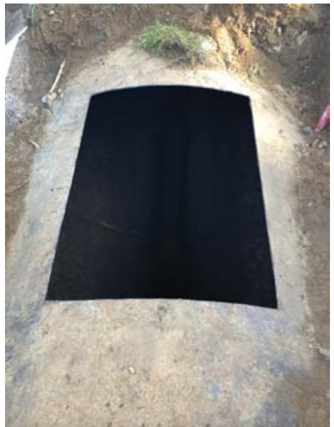
Fig. 2: Excavated manhole access
