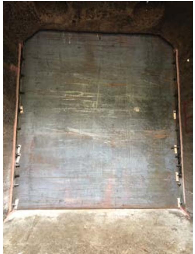
Fig. 1: Temporary safety bulkhead
