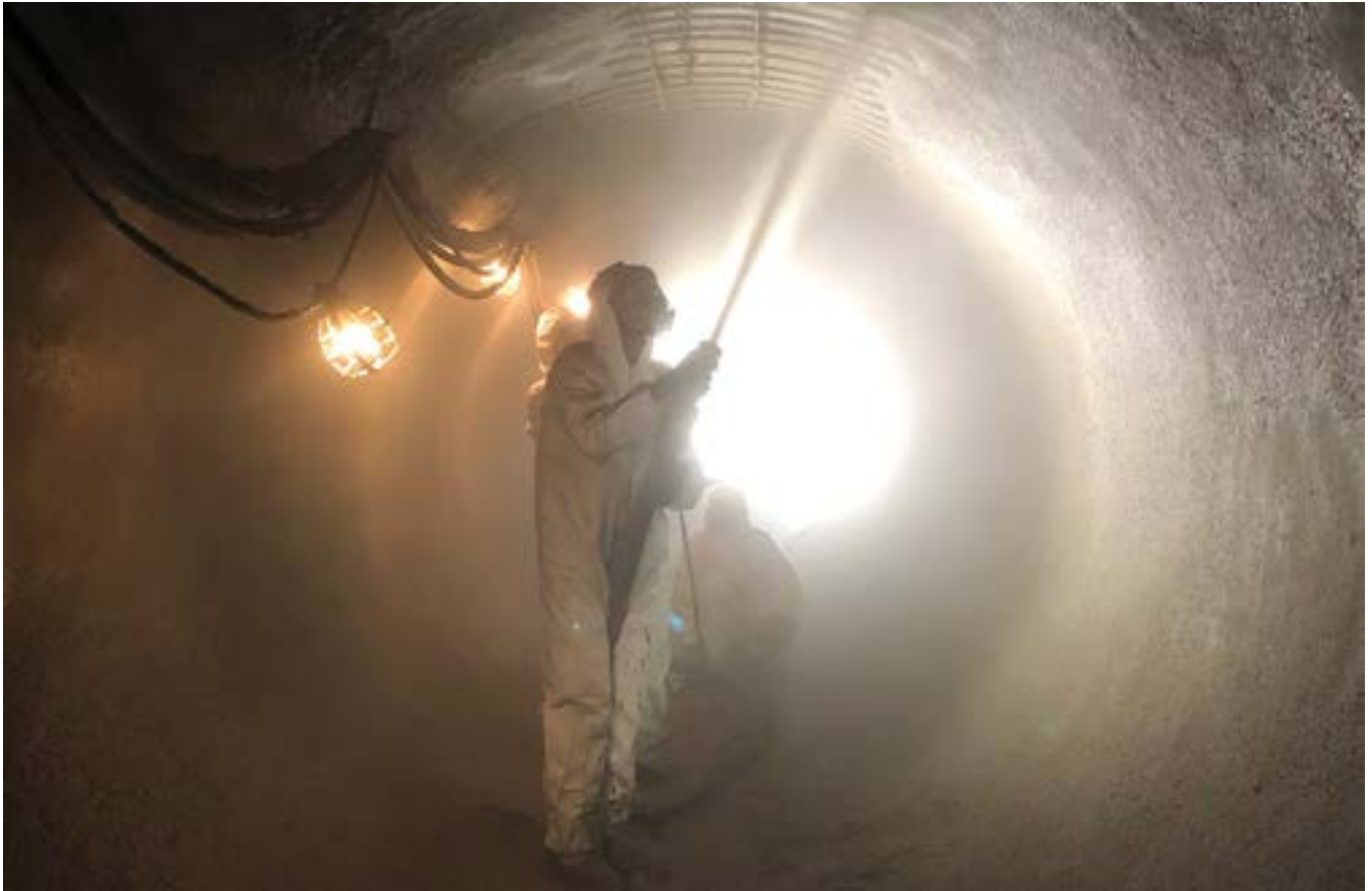
Fig. 5: Falls Village Penstock shotcrete
