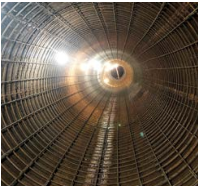
Fig. 4: Reinforcing bar installed
