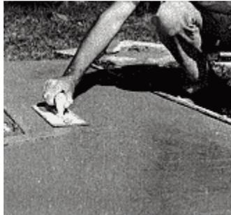
8. Once the concrete has set up, swing the trowel in the same circular pressing and polishing motion that was used in floating. Continue working until the surface is smooth and dense. You may wish to allow the concrete to continue to harden and then trowel once more for the densest possible finish. After troweling, redo edges and grooves.
