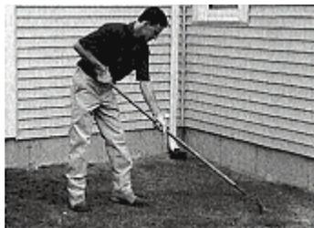
2. Remove the sod and soil to the desired depth. Remember to account for the width of the forming lumber.
