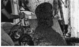
**2.** Dampen the subgrade before making the pour. Note the use of a splash board to help direct the flow.
