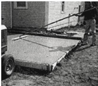
**6.** Cut the concrete away from the forms by running an edging tool along the forms to compact the slab edges.
