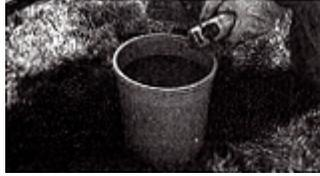
3. Mix thoroughly until the concrete is uniform in color. Add water as needed to achieve consistency.
