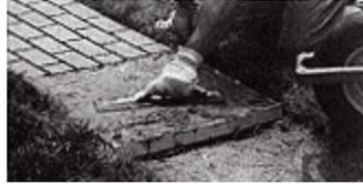
**3.** Remove the mold promptly, and smooth the concrete edges with a trowel until the desired appearance is obtained.
