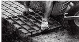
**4.** Place the mold adjacent to the completed section and continue this process until your project is completed. By alternately rotating the Walk Maker® mold one quarter turn each time, a variation in the pattern is achieved.
