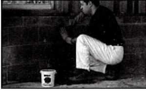
**5.** Beginning at the top, press the cement into the cavity with your fingers. Maintain pressure for a few minutes or until the cement sets and the leak stops.
