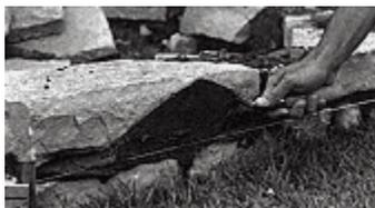
**7.** Rake out the joints to a depth of  $\frac{1}{2}$ " after the mortar has set slightly; this will highlight the stone edges. If a slicker jointer is not available for this, use a wooden dowel or small stick.
