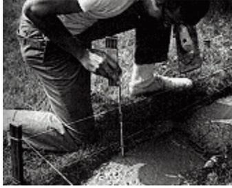
**4.** Butter the head joints of the stones before setting them in place. Once the first course has been laid, spread a layer of mortar on top of the stones and begin laying the second course.
