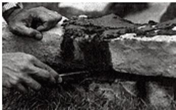
8. After the second course has been laid, it will probably be necessary to raise the mason's line in order to check that the planter is straight. Because the face of stone is not smooth like brick, the stone is plumbed "bump to bump."
