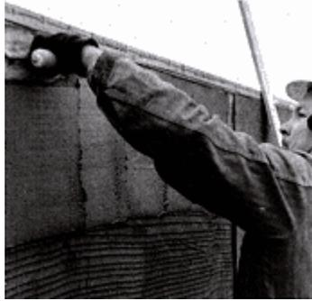
4. Screed the brown coat evenly by running the edge of a straight board over the brown coat and smoothing out the high and low spots.
