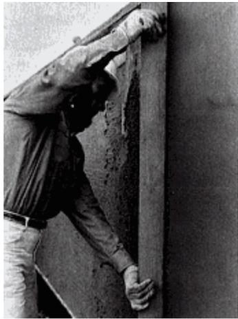
6. Moist-cure the brown coat for 2 days, and then air cure for 5 additional days before applying the finish coat.
