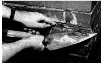
**3.** In most cases, joints are filled flush to the wall face, then slightly depressed with the jointer and brushed clean. If concave or V joints were used in the original work, strike with the proper tool for these finishes after the repointing is done and before the mortar gets too hard to work.
