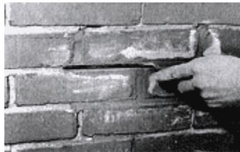
**4.** To decrease the possibility of cracking or sagging in extremely deep joints, fill in about half of the joint depth, wait until the mortar is thumbprint hard, and then repoint the remainder of the joint.
