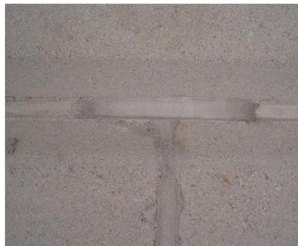
**Leading edge discoloration of a mortar patch – over tooling**
